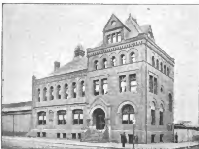
RAILROAD BRANCH, Y. M. C. A., MADISON AVENUE AND 45TH STREET.
